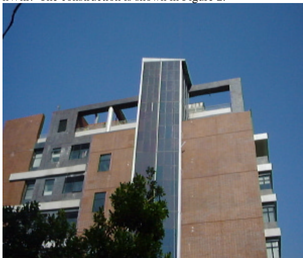
Figure 2. The constructed PV façade in HKU
